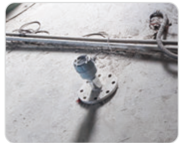
Feeding plant Corn storage tank detection
