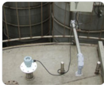
Oil Factory Soybean oil level detection
